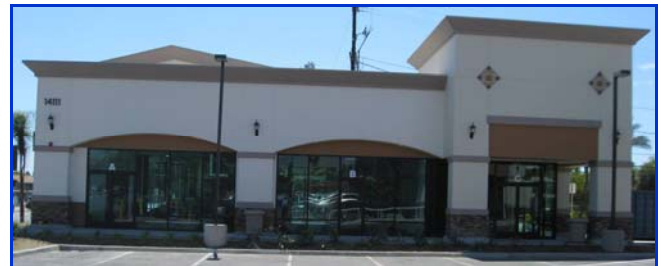
North Elevation of Pad Building
